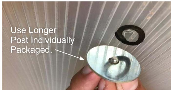
Using longer Chicago screw set, attach a metal washer on one side and hand screw together through the washer ► through the panel ► and attach other side of screw. Orientation of Chicago screw does not matter. No magnet on this step.
